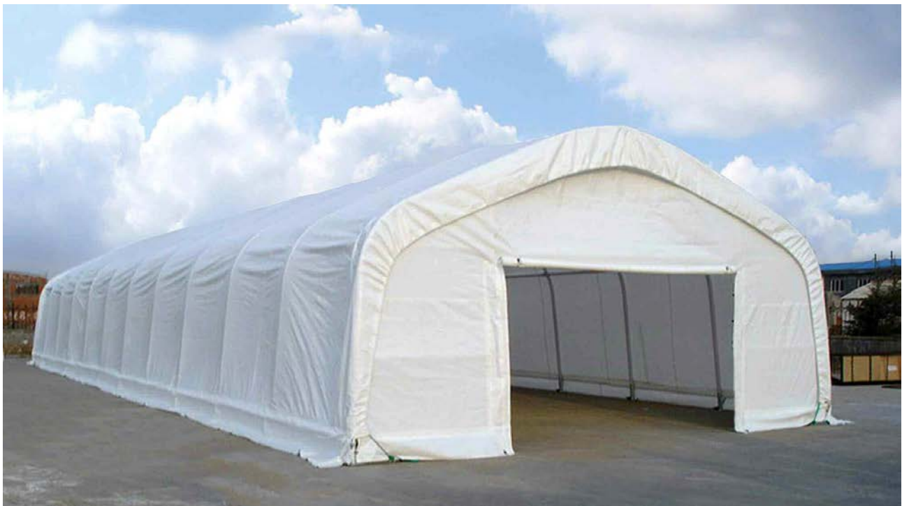
Figure 2-4 Example of the mobile enclosure for IBA maturation
